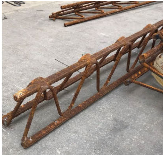
Photo 1: Typical Temporary Reinforcement Trusses prior to the bottom chords being cast into the 130mm thick precast deck panel.
