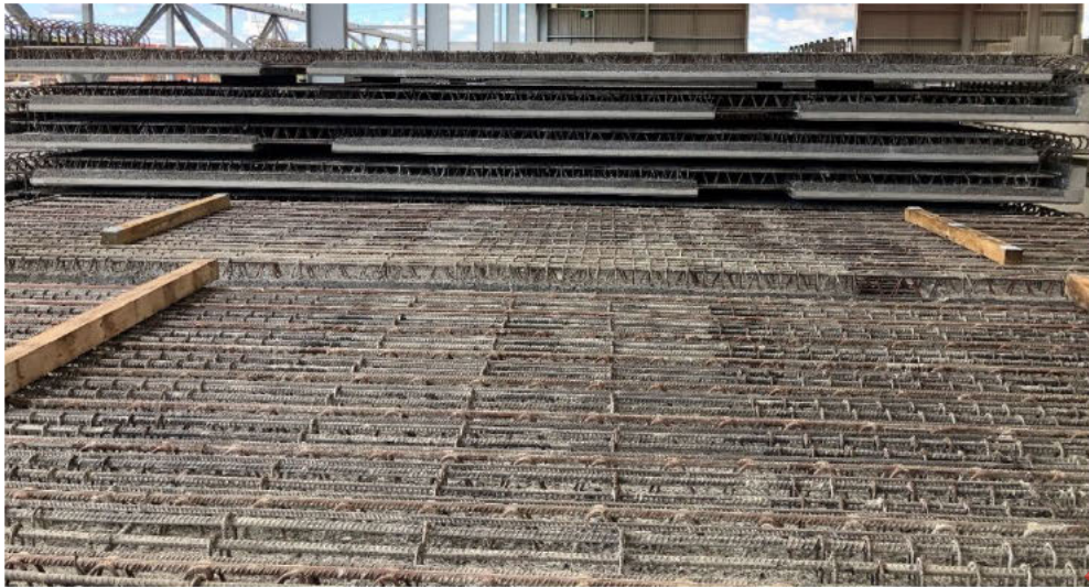
Photo 3: Typical outer precast deck panels stacked and ready to be transported to the Okahu site.
