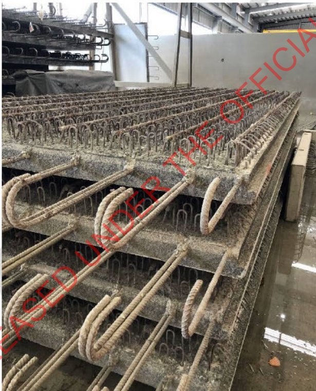
Photo 2: Typical centre precast deck panels stacked and ready to be transported to the Okahu site.
