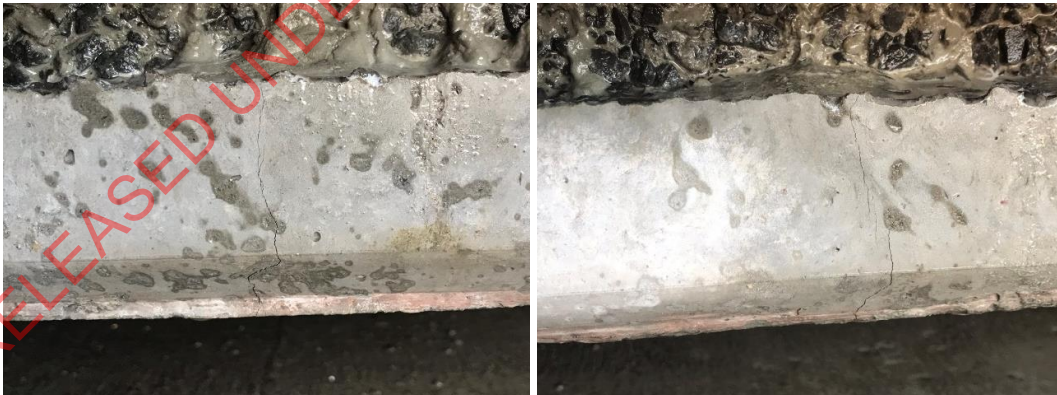
Figure 2.8: Cracking observed at ULS
