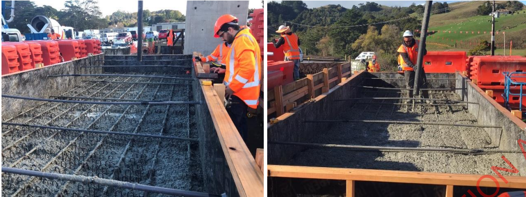
Figure 2.6: ULS load testing in progress
