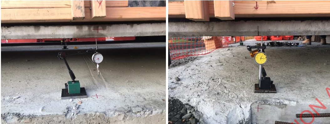
Figure 2.3: Dial Gauges setup at mid-span and near end of cantilevers
