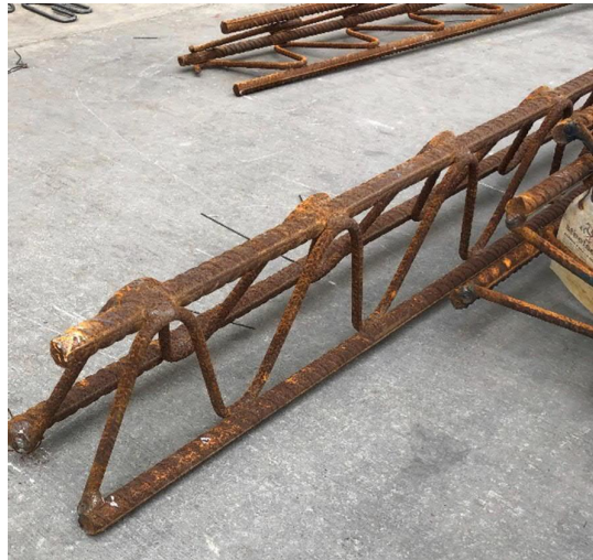
Photo 1: Typical Temporary Reinforcement Trusses (TRT)
