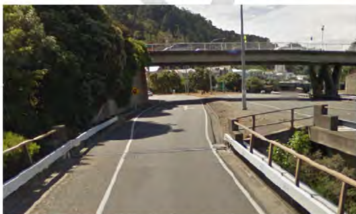
Figure 8.4: Tinakori Road Off-Ramp Bridge – Trailing Approach Barriers and End Terminals
