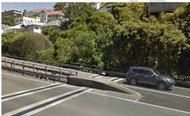
Figure 9.7: Shell Gully Overbridge (Northbound) – Edge Barrier Trailing End Terminal
