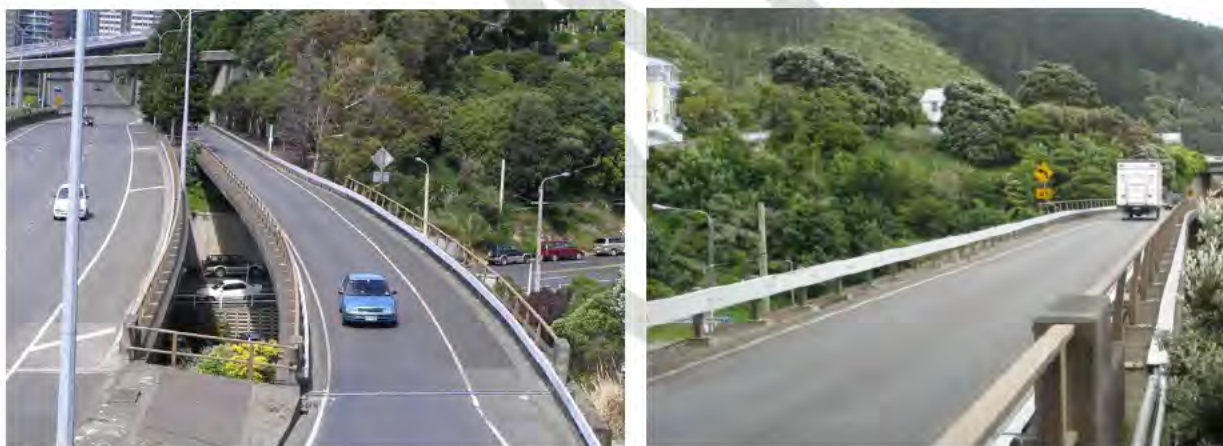
Figure 8.1: Tinakori Road Off-Ramp Bridge – Barrier Systems
