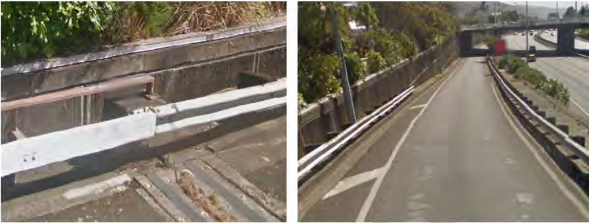
Figure 5.5: May Street On-Ramp – Trailing Transition and Barrier System
