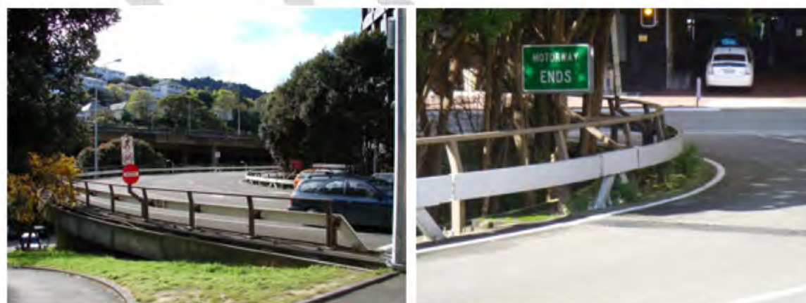
Figure 10.3: Terrace Off-Ramp Bridge – Trailing End Barrier Terminals
