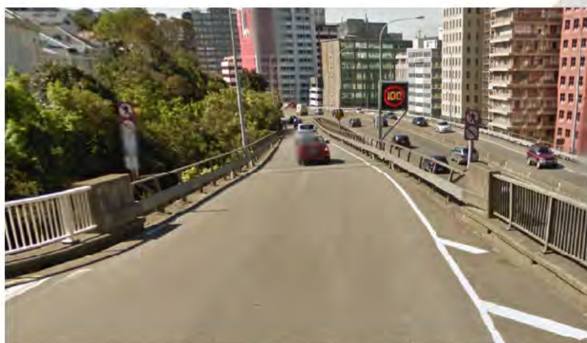
Figure 11.1: Clifton Terrace On-Ramp Bridge – Leading Approach Barriers
