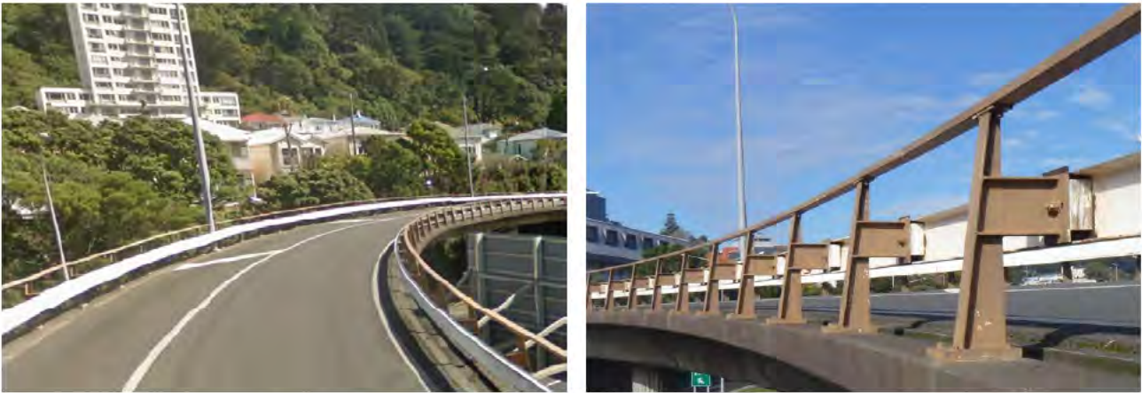
Figure 5.1: May Street On-Ramp – Barrier System
