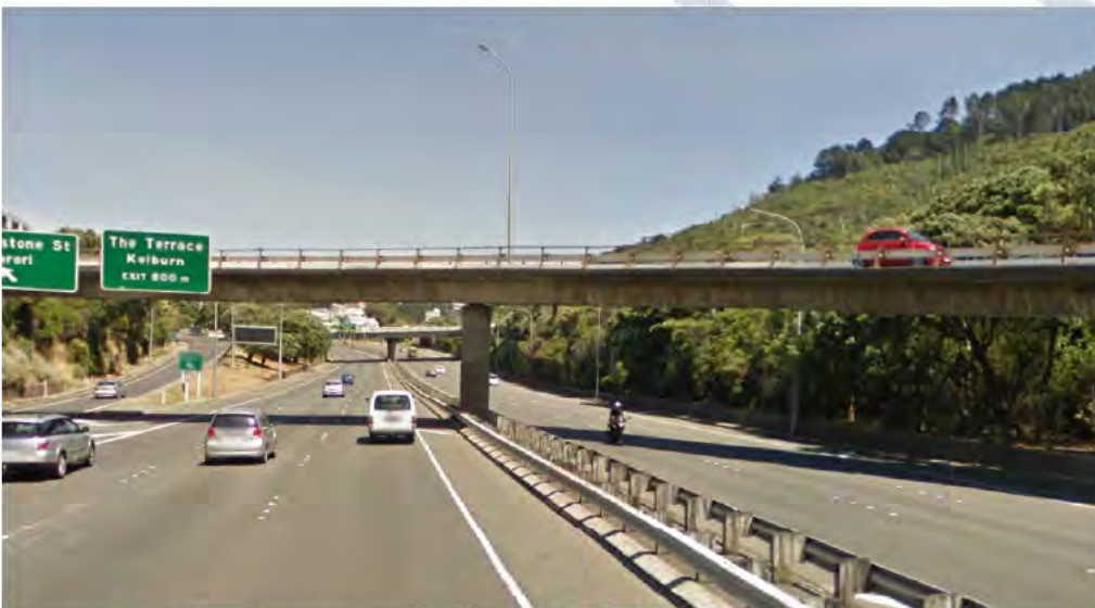
Figure 5.2: May Street On-Ramp – Bridge Structure and WUM
