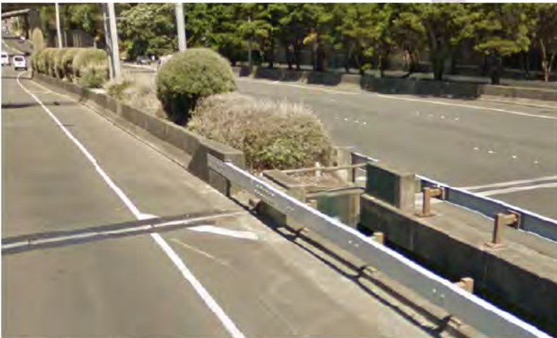
Figure 6.7: Bowen Street Overpass (Southbound) – Median Barrier Trailing Transition System
