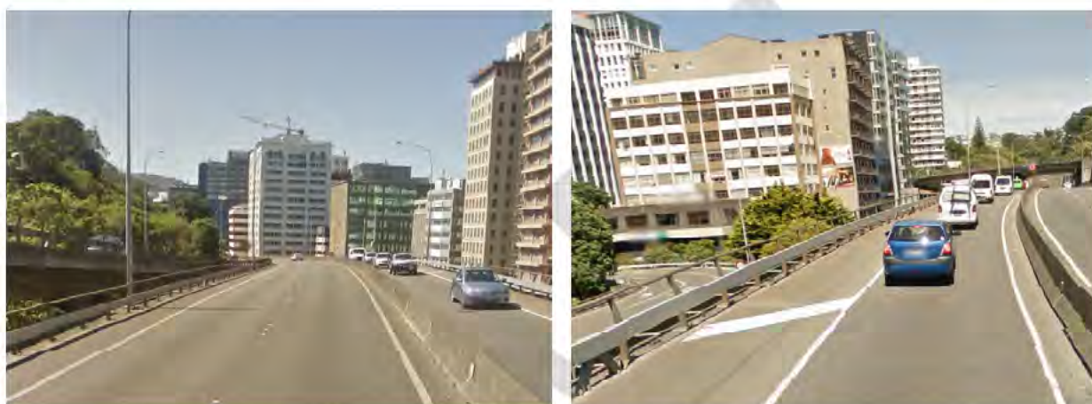
Figure 9.1: Shell Gully Overbridge – Edge Barrier and Median Barrier
