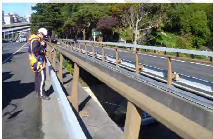
Figure 7.2: Bowen Street Overpass (Northbound) – Top Handrail
