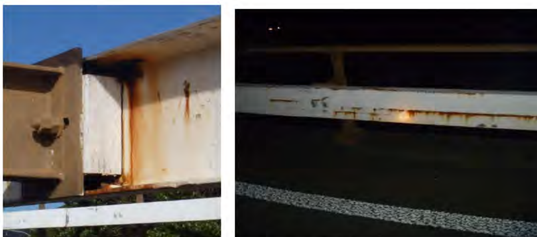
Figure 5.6: Corrosion on the Steel Channel Rail
