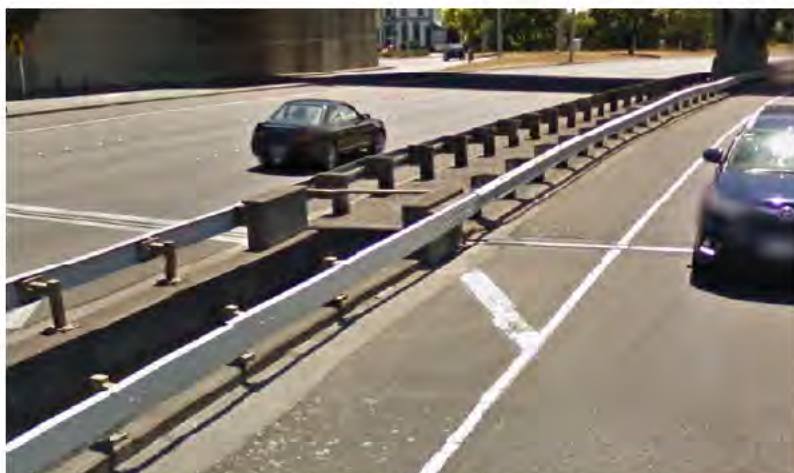
Figure 6.8: Bowen Street Overpass (Southbound) – Median Barrier Leading Transition Approach
