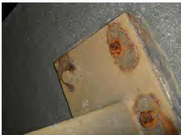
Figure 8.5: Corrosion of Baseplate Hold-down Bolts
