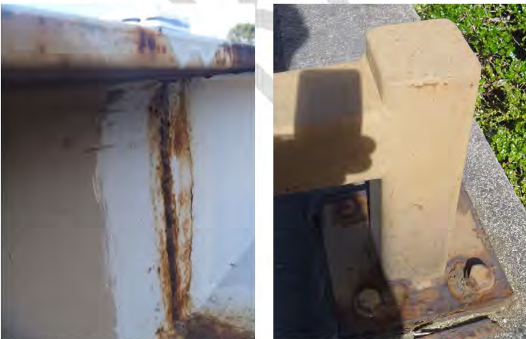
Figure 6.10: Corrosion at Welded Connection in the Rail and around Post Baseplate
