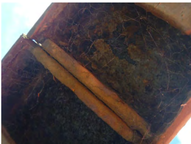
Figure 7.7: Corrosion on the Underside of the Top Handrail
