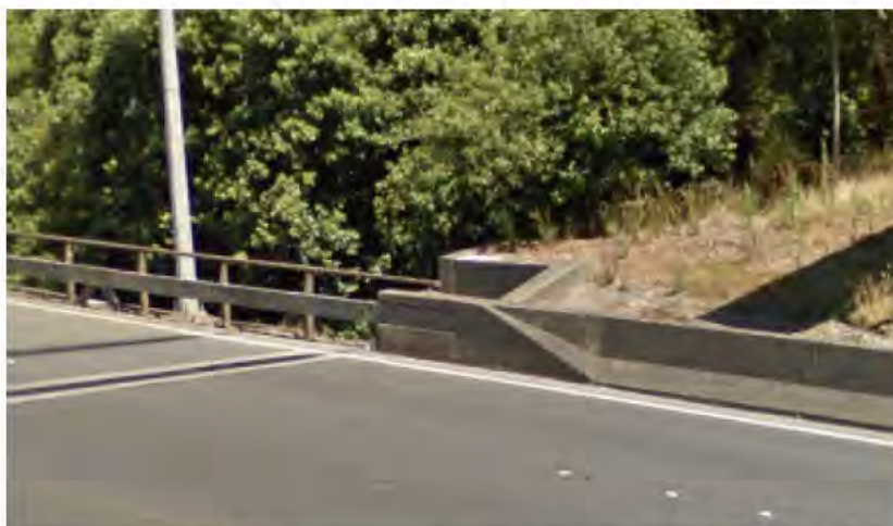
Figure 11.3: Clifton Terrace On-Ramp Bridge – Edge Barrier Trailing Approach
