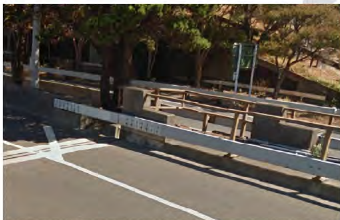
Figure 7.4: Bowen Street Overpass (Northbound) – Edge Barrier Leading Approach
