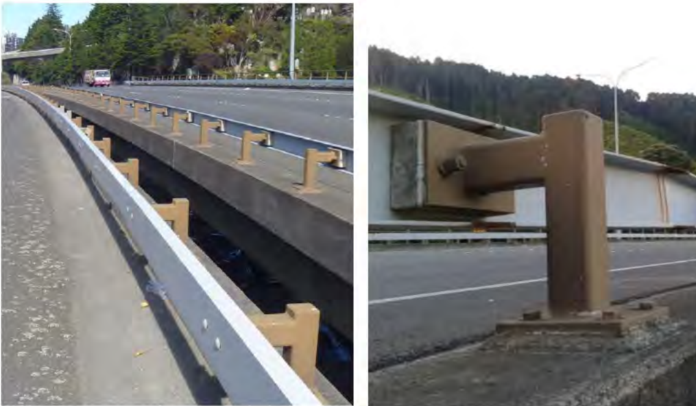
Figure 6.4: Bowen Street Overpass (Southbound) – Median Barrier System
