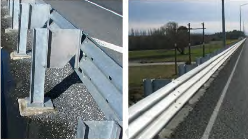
Figure 3.3: TL-4 Thrie-beam (with Modified Blockout) Barrier System
