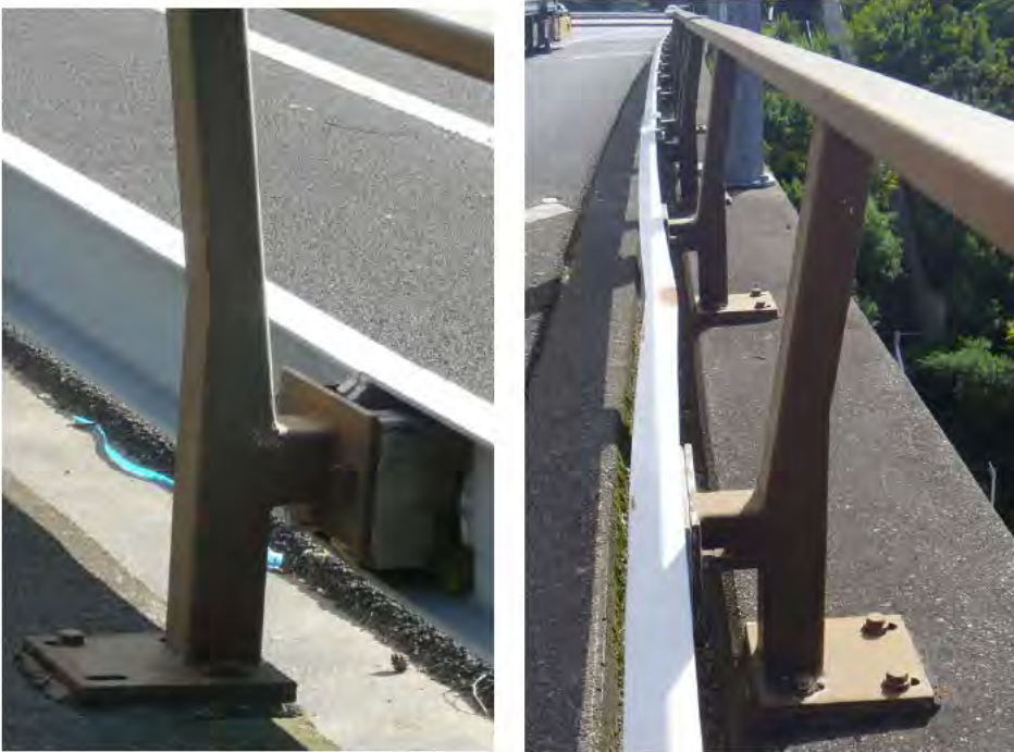
Figure 6.1: Bowen Street Overpass (Southbound) – Edge Barrier Post
