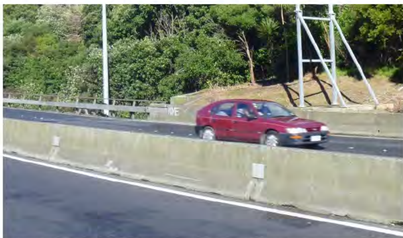
Figure 8.7: Shell Gully Overbridge (Northbound) – Median Concrete Barrier
