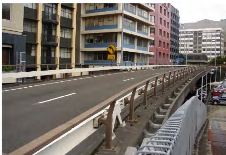
Figure 10.1: Terrace Off-Ramp Bridge – Barrier Post and Rail
