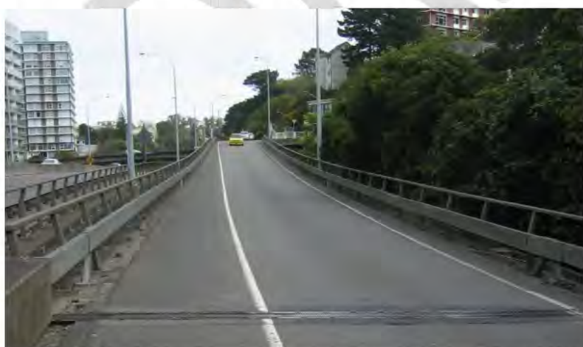
Figure 11.2: Clifton Terrace On-Ramp Bridge – Steel Channel Rail Barrier System
