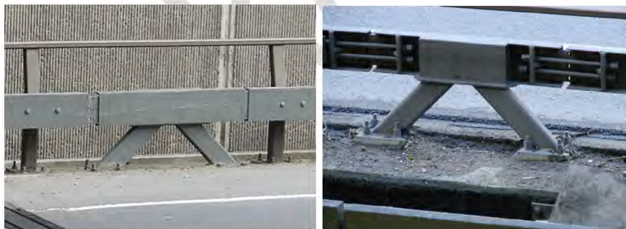
Figure 9.3: Shell Gully Overbridge – Rail Anchorage to Bridge Deck
