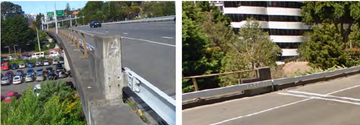
Figure 6.6: Bowen Street Overpass (Southbound) – Concrete Anchor Block
