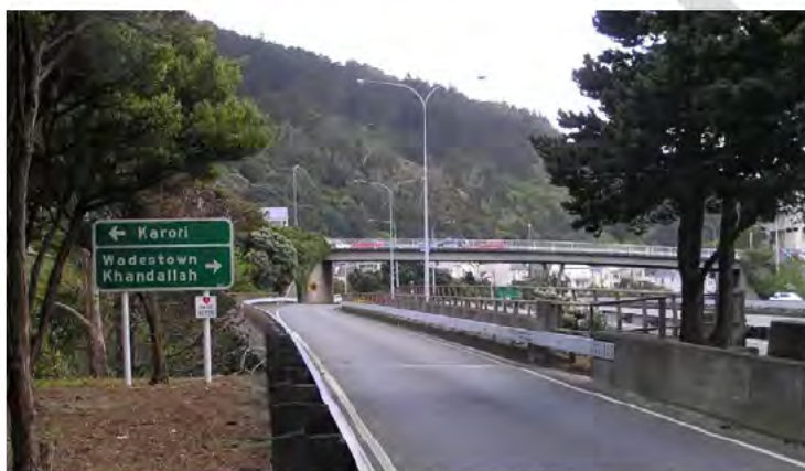
Figure 8.3: Tinakori Road Off-Ramp Bridge – Leading Approach Barriers
