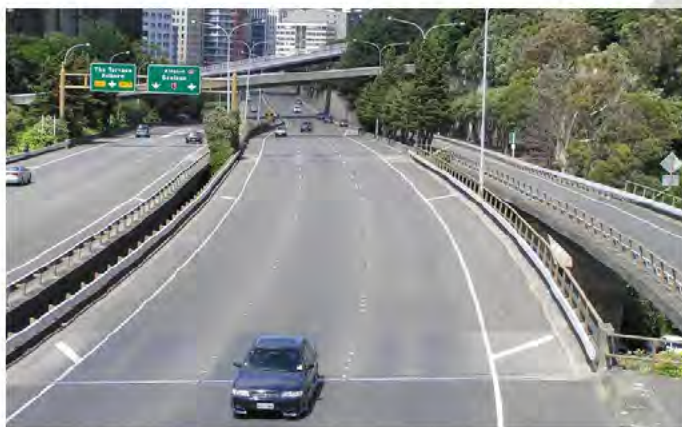
Figure 7.1: Bowen Street Overpass (Northbound) – Barrier System
