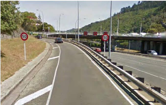
Figure 4.2: Murphy Street Off-Ramp – Edge Barrier
