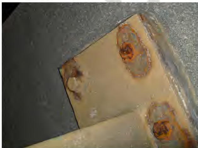
Figure 8.5: Corrosion of Baseplate Hold-down Bolts
