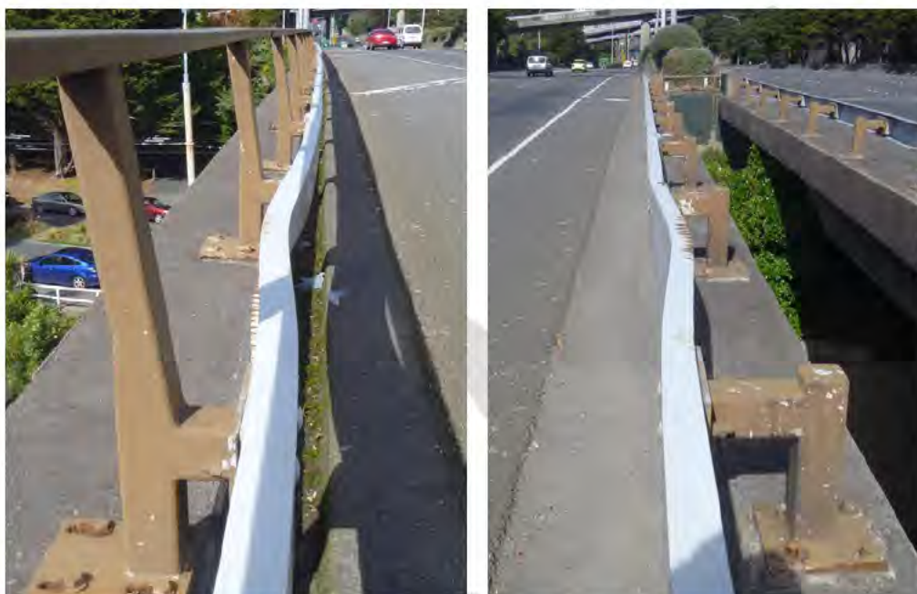
Figure 6.11: Examples of Barrier Damage from Vehicle Impacts
