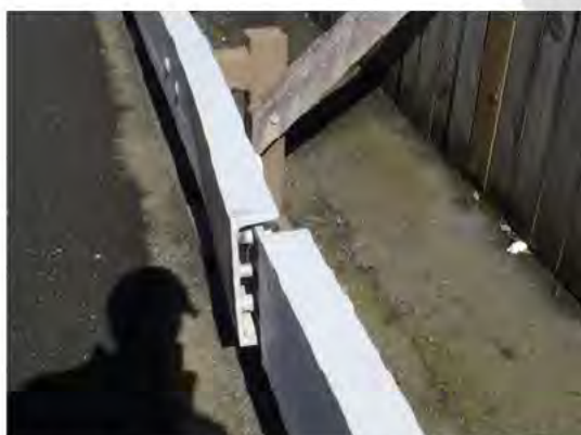
Figure 10.5: Misaligned Rail due to a Vehicle Impact
