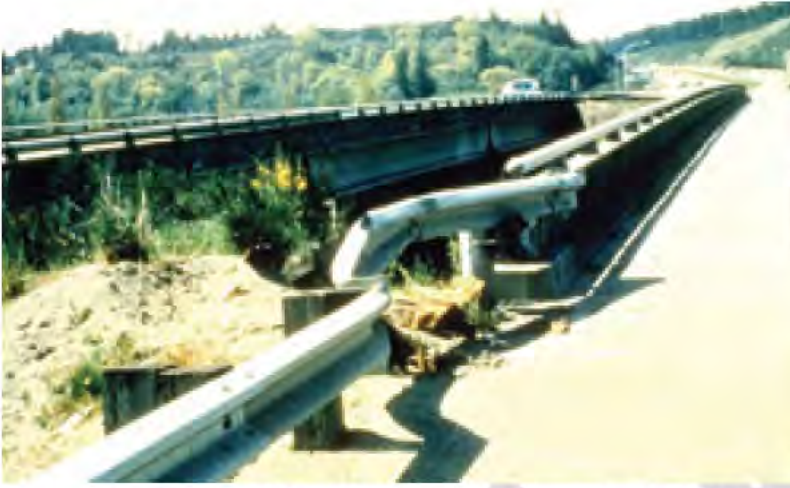
Figure 6.9: Example of Vehicle Pocketing (source – US Department of Transportation)
