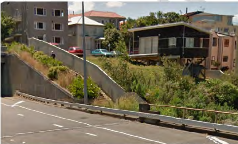
Figure 6.5: Bowen Street Overpass (Southbound) – Edge Barrier Leading Approach
