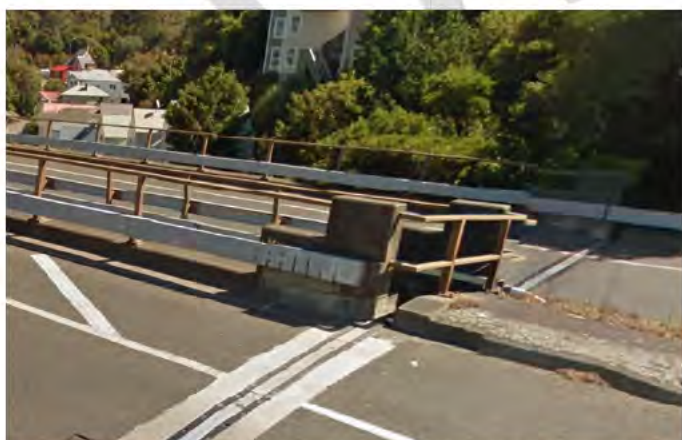
Figure 7.5: Bowen Street Overpass (Northbound) – Barrier System Trailing Terminal
