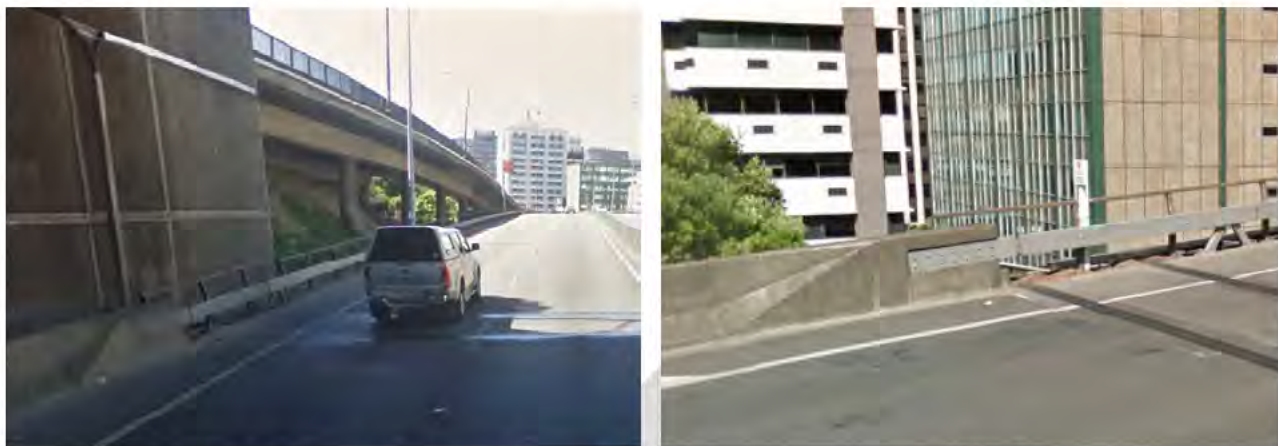
Figure 9.6: Shell Gully Overbridge (Northbound) – Leading Approach Barriers
