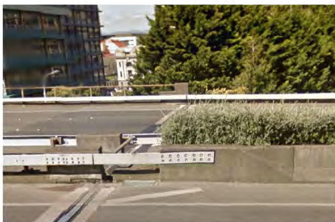
Figure 7.3: Bowen Street Overpass (Northbound) – Median Barrier Leading Approach
