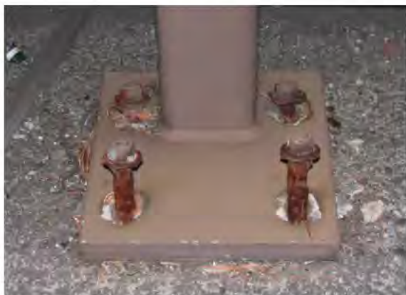
Figure 10.4: Corroded Hold-down Bolts
