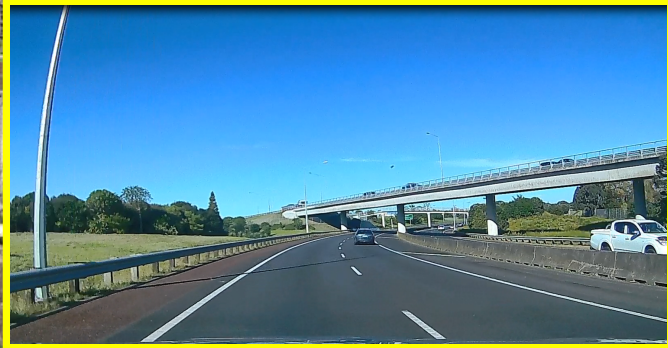
Left shoulder widening by reallocating space from the right shoulder
