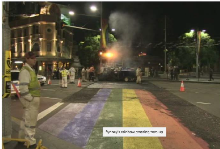
PHOTO: Sydney's rainbow crossing is covered in asphalt.
