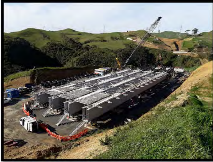
Photo Above: Bridge 20 Launch Nose
