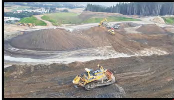
Photo Above: Cut 42 processing material to send to the RSE/MSE Walls
