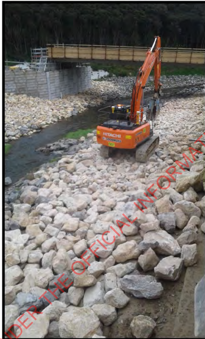
Photo Above: Pauatahanui Stream Diversion – Bridge 14 in background
