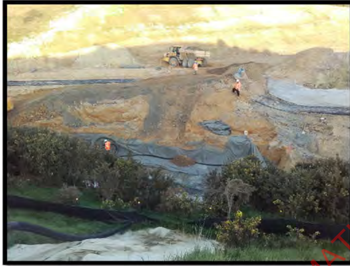
Photo Above: 15815 Muck Out
