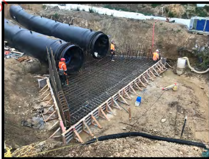
Photos Above: 21310 Inlet – Slab ready to be poured.
