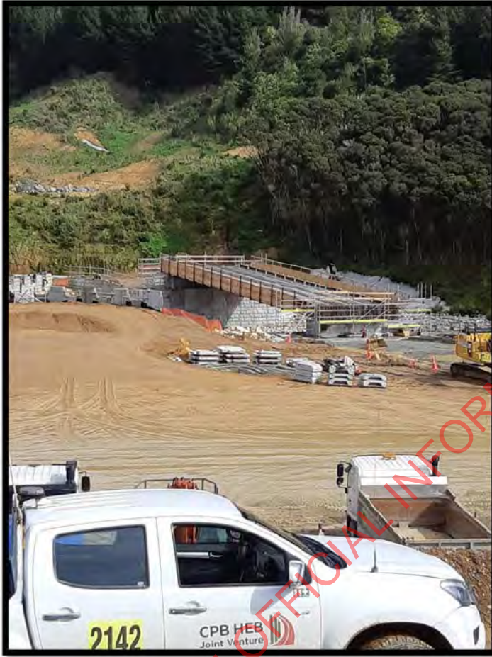
Photo Above: Bridge 14 Beam Complete
