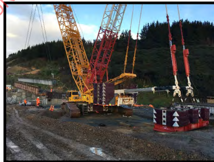
Photo Above: Bridge 14 Beam Placement
