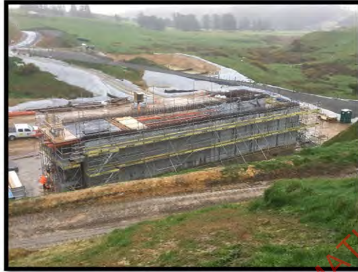
Photo Above: Bridge 11 Roof
