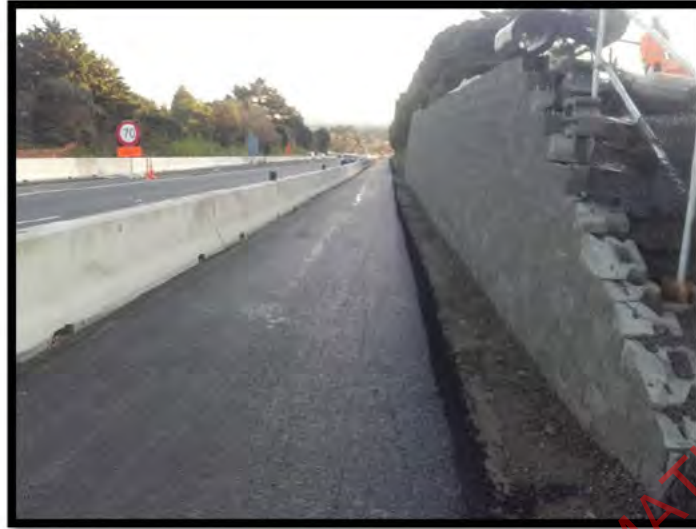
Photo Above: Bridge 25 and temporary widening
