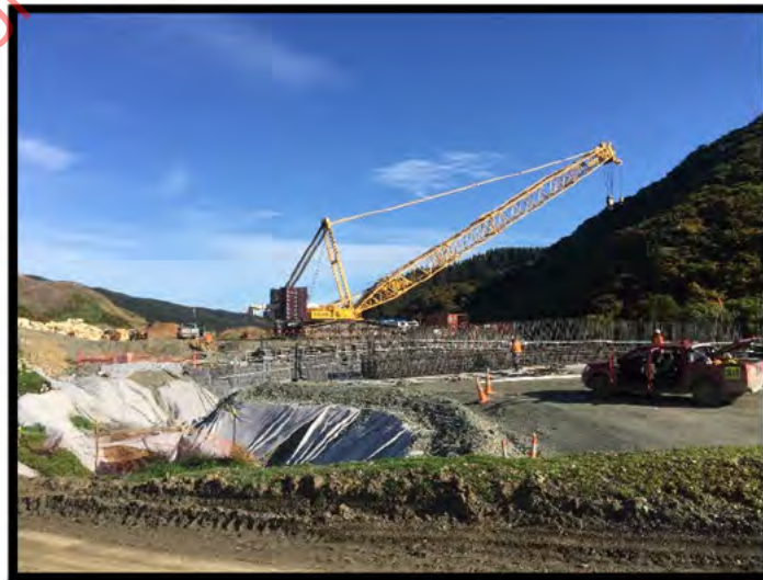
Photo Above: Bridge 4 Abutments
