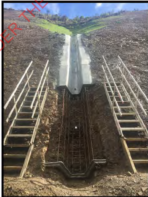
Photo Above: Cut chute at Wainui Saddle
