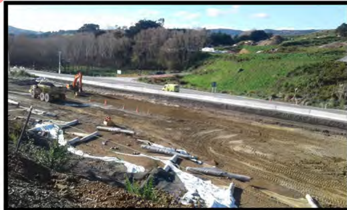
Photo Above: Foundation Treatment beside SH58
