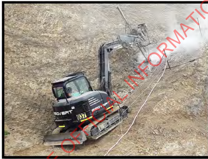
Photo Above: Cut 23 Swale Anchors
