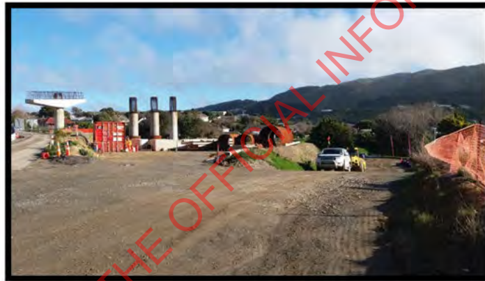
Photo Above: Bridge 27A access around bridge 27 abutment A
