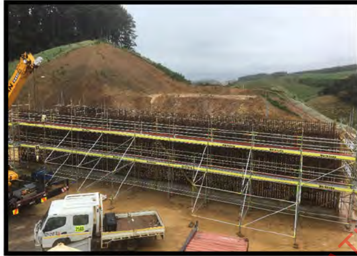
Photo Above: Bridge 18A Walls
