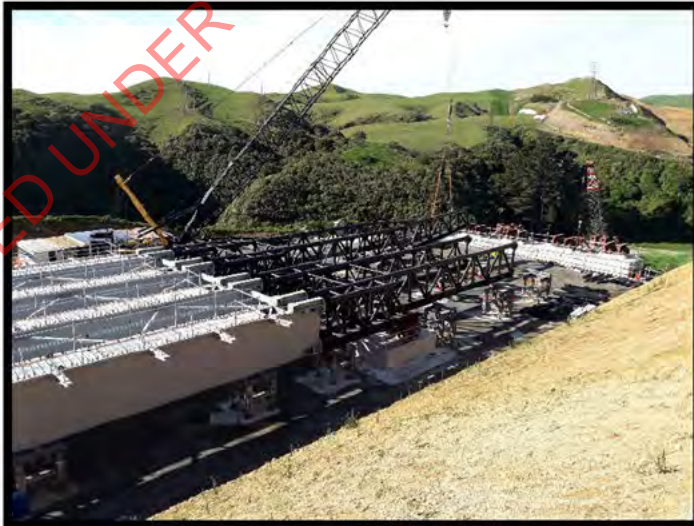
Photo Above: Bridge 20 Launch Nose
