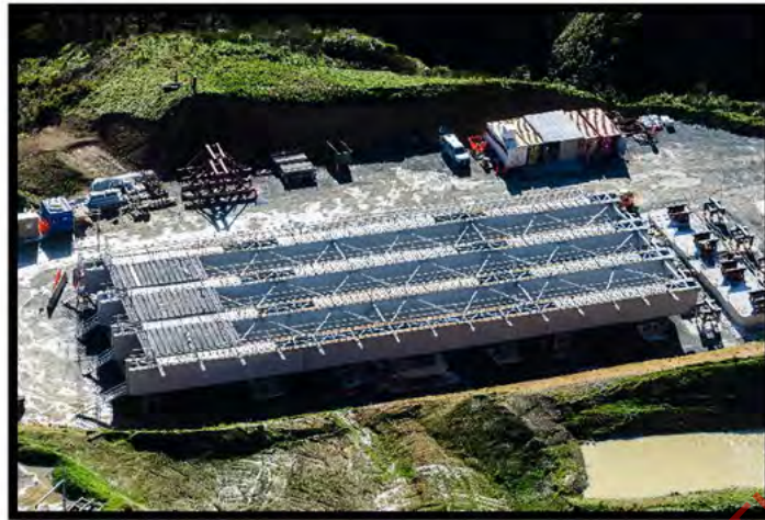
Photo Above: Bridge 20 – Launch Yard
