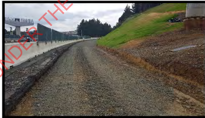
Photo Above: Subgrade CLR2
