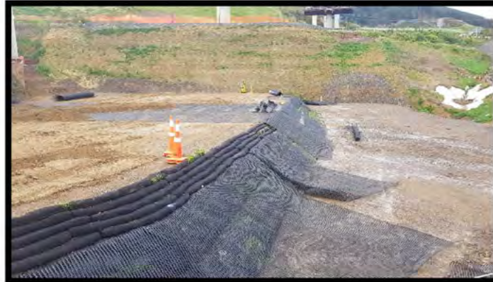
Photo Above: Bridge 27A
