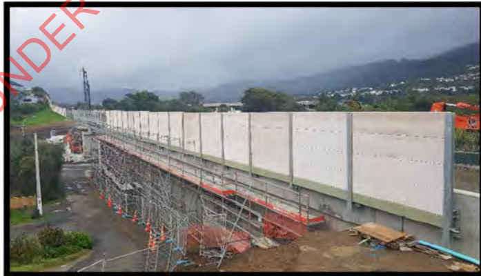
Photo Above: Bridge 26
