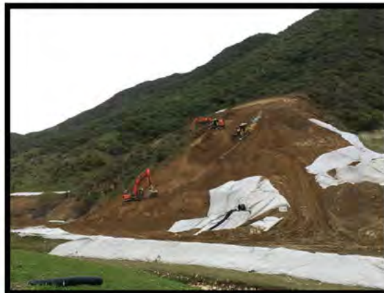
Photo Above: B1 Lime drying fill Te Puka 5
