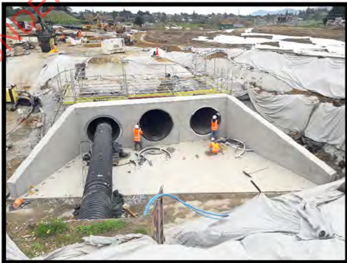
Photo Above: Headwalls CH1850
