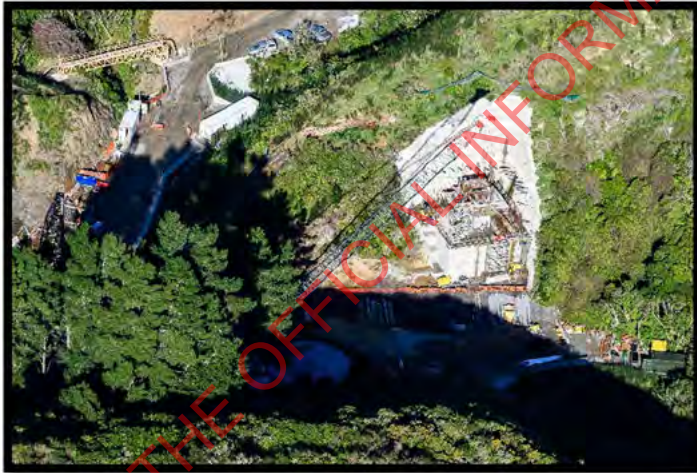
Photo Above: Bridge 20 – Pier 2
