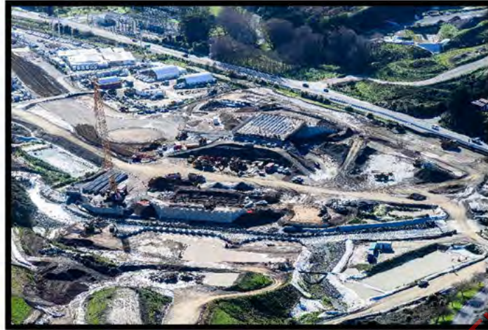
Photo Above: SH58
