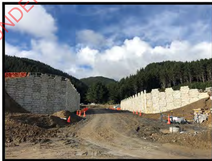
Photo Above: Bridge 2
