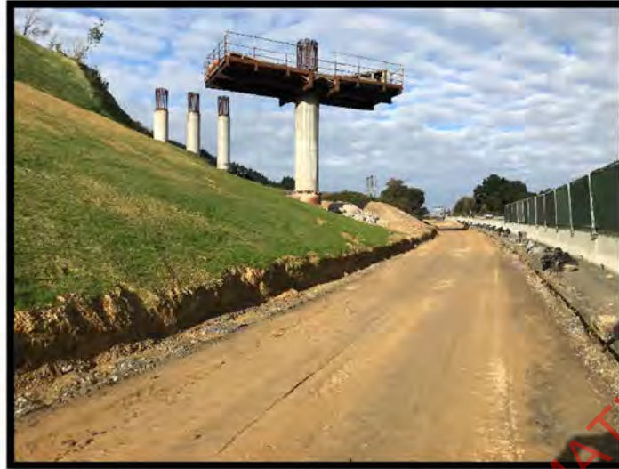
Photo Above: CLR2 SH1 SB widening works - construction platform
