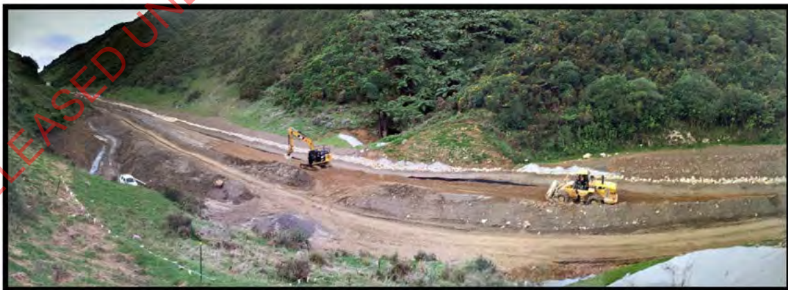
Photo Above: Ch. 6700
