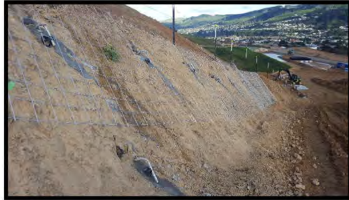
Photo Above: Stabilisation works to Cut 42
