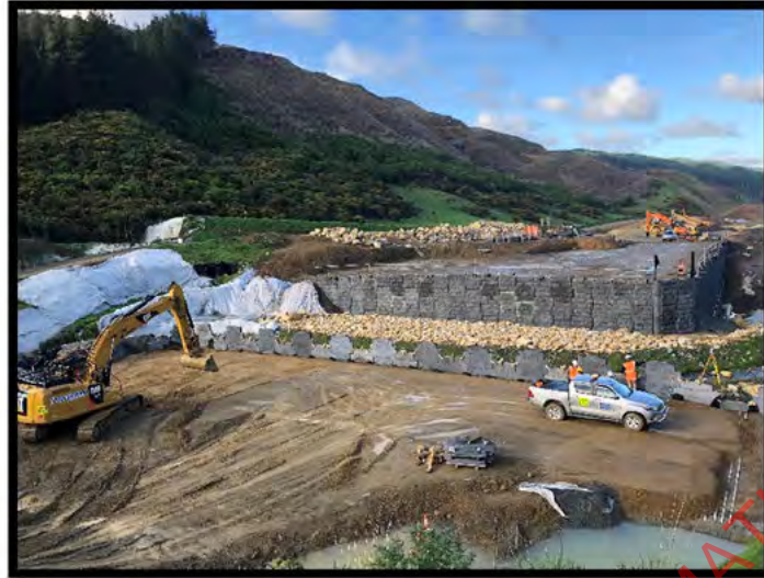
Photo Above: Bridge 4
