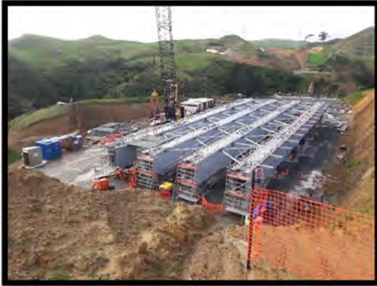
Photos Above: Bridge 20 Superstructure – Deck Panels
