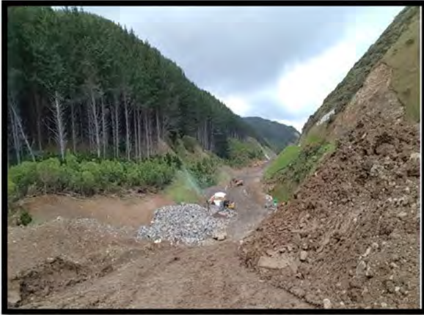
Photo Above: B1 Te Puka 5 Stream Diversion
