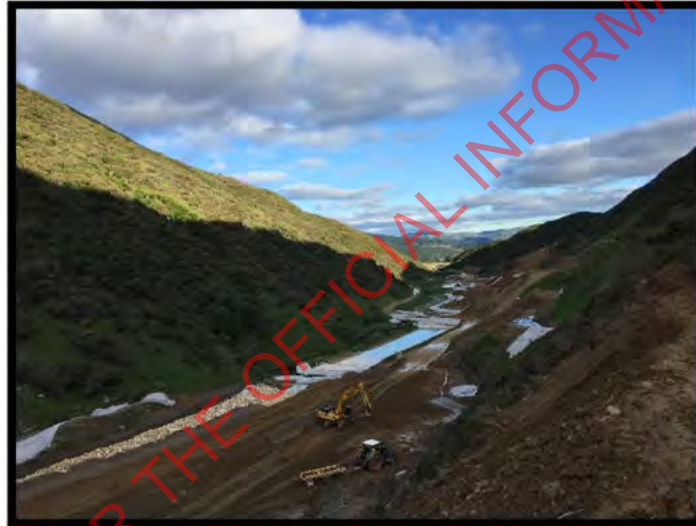
Photo Above: B1 Te Puka 5 Stream Diversion
