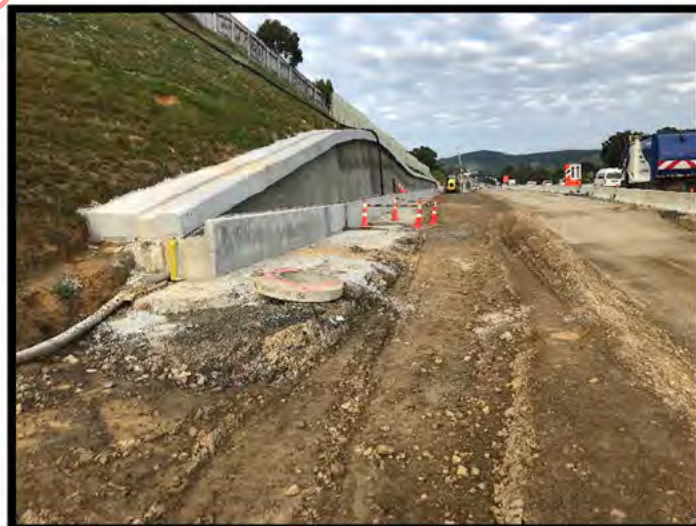
Photo Above: Retaining Wall 4 capping beam and precast panel foundation complete
