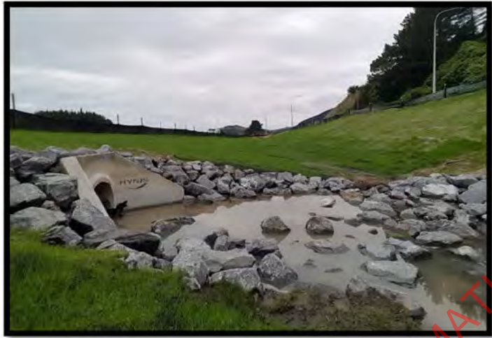
Photo Above: A1 Coast Rd Swale drain Fill 1 batter Ch 850 - 600
