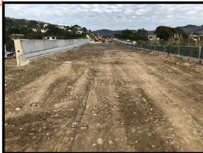
Photo Above: Bridge 26 - Northern approach embankment
