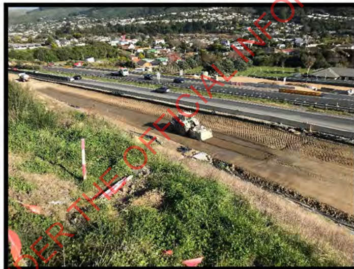
Photo Above: Cut 45 - Construction Platform
