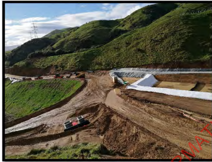
Photo Above: Bridge 19
