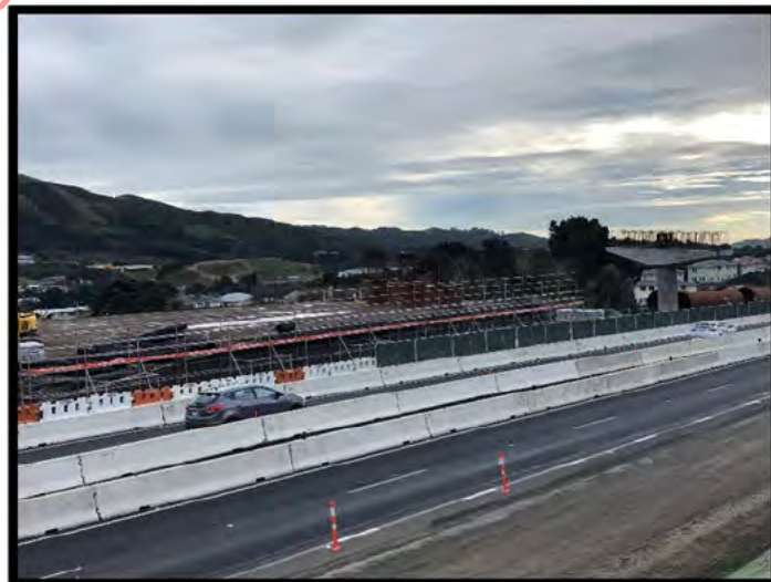
Photo Above: Bridge 25A - SH1
