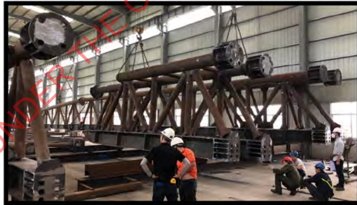
Photo Above: Bridge 20 Launch Nose
