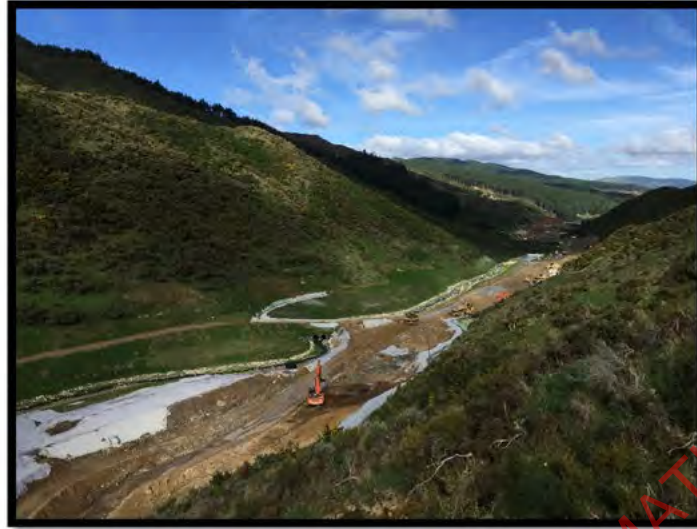
Photo Above: B2 Fill 5 Ch. 7400 to 7700 foundation treatment
