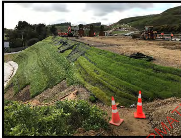
Photo Above: Bridge 25 - Abutment A MSE and RSE Embankment Construction
