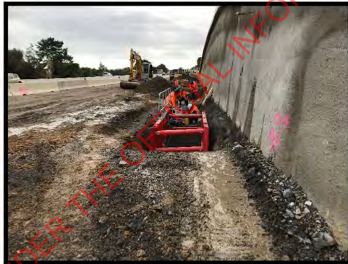
Photo Above: Cut 47 - Longitudinal Drainage Installation
