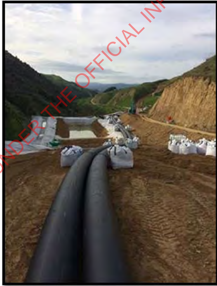
Photos Above: Temp Bulk Water Relocation - BR19
