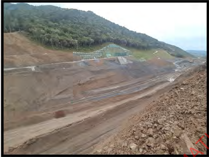
Photo Above: B1 Cut 5C fourth batter shotcrete
