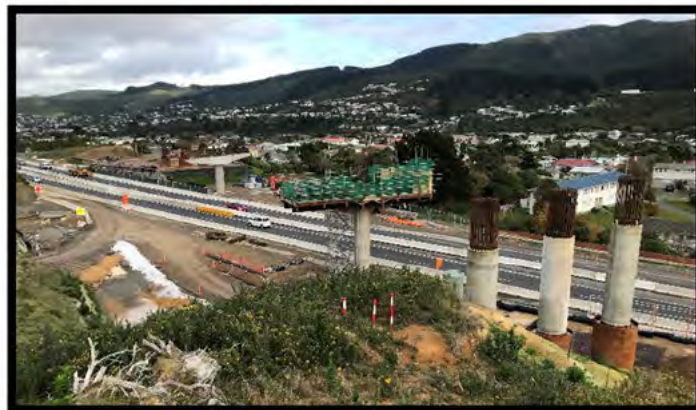
Photo Above: Bridge 25 - View looking South
