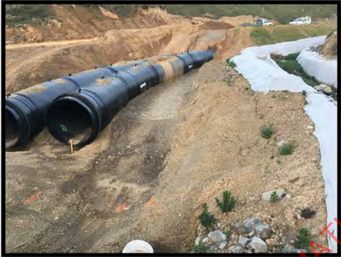
Photo Above: 21310 Culvert
