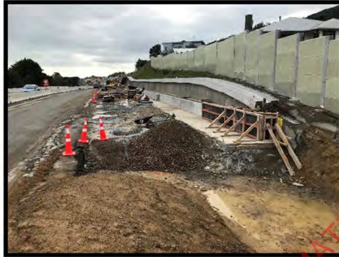
Photo Above: RW4 Capping Beam and Facing Panel Foundation Construction
