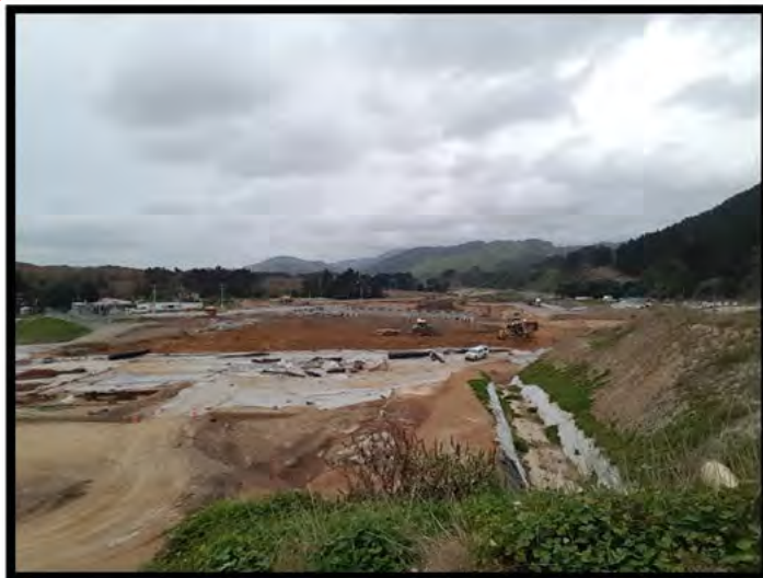
Photo Above: A2 Fill 2B and 2A foundation treatment
