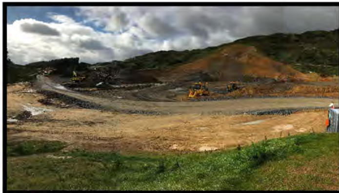
Photo Above: Cut 42 - Material Processing
