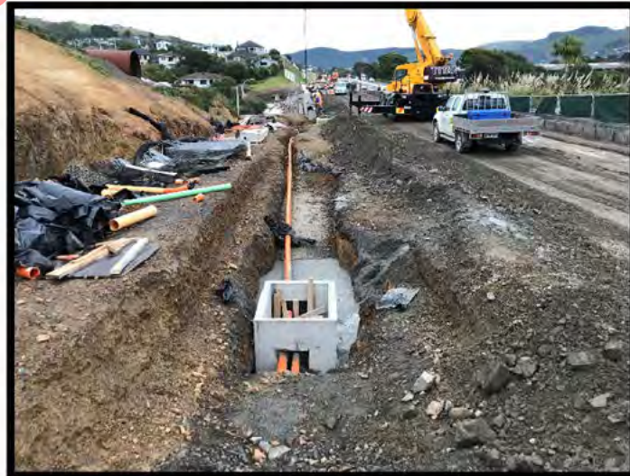
Photo Above: ITS Installation - Cut 45
