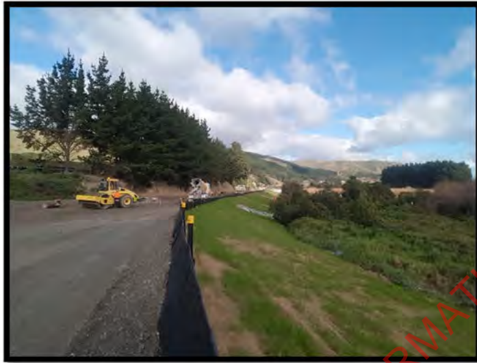
Photo Above: A1 Coast Rd Stabilised Fill Batter Ch. 200 - 500
