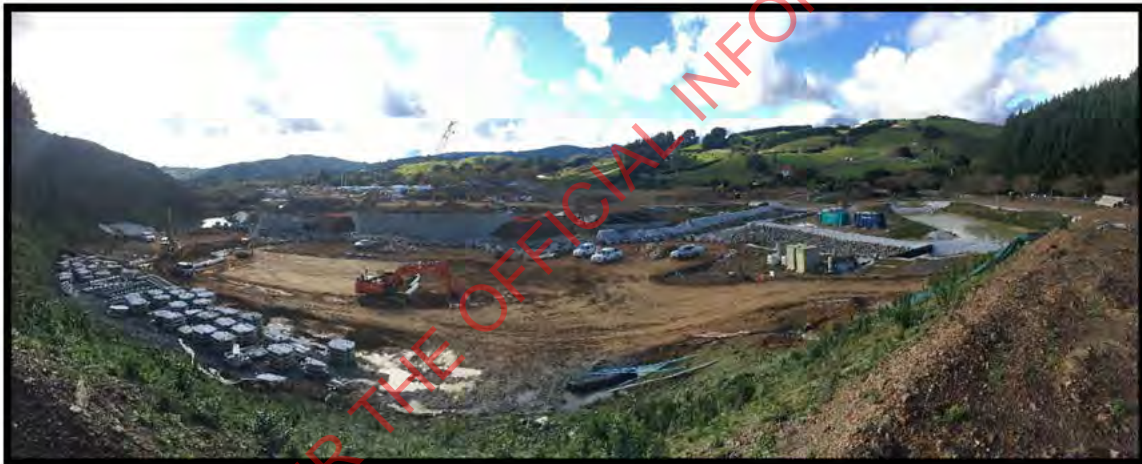
Photo Above: SH58
