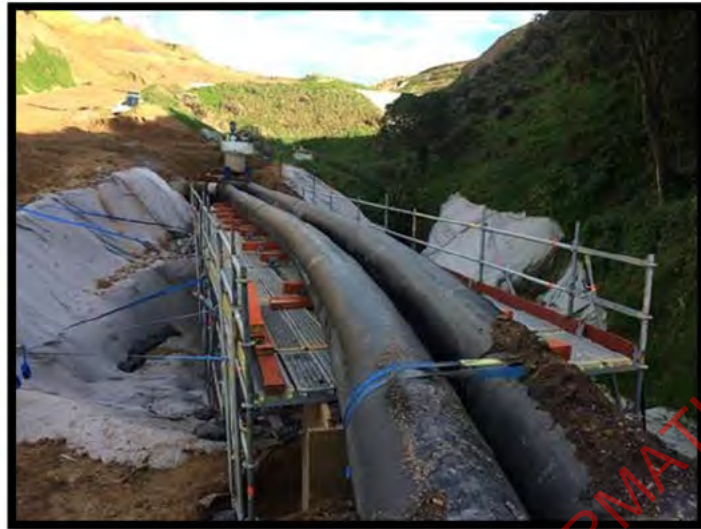
Photo Above: Temp Bulk Water Relocation - BR19
