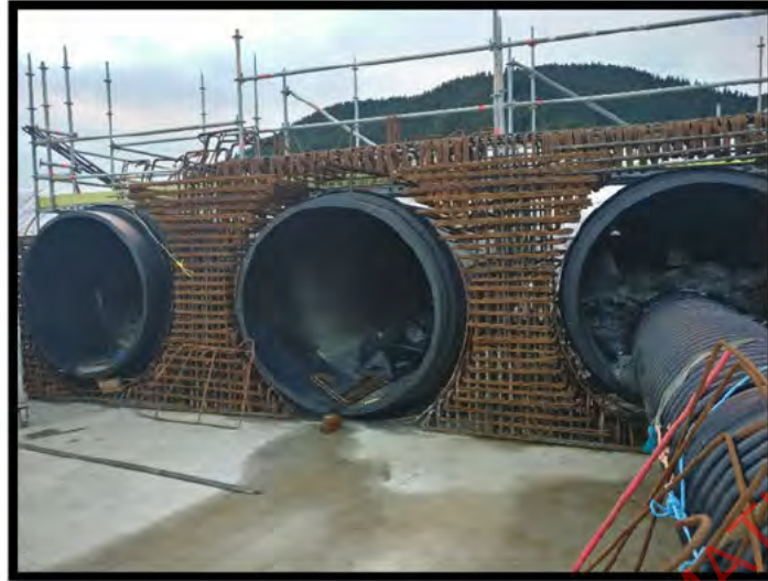
Photo Above: CH1850 - Outlet
