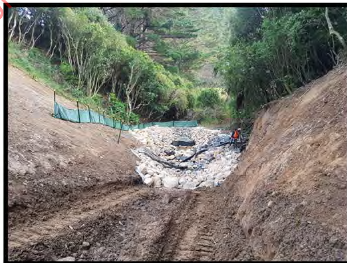
Photo Above: Stiling Basin
