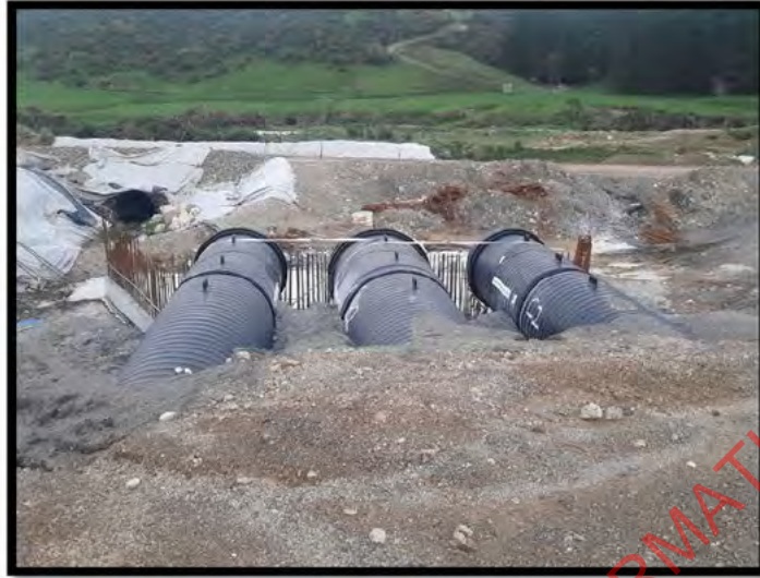
Photo Above: 9040 Culvert
