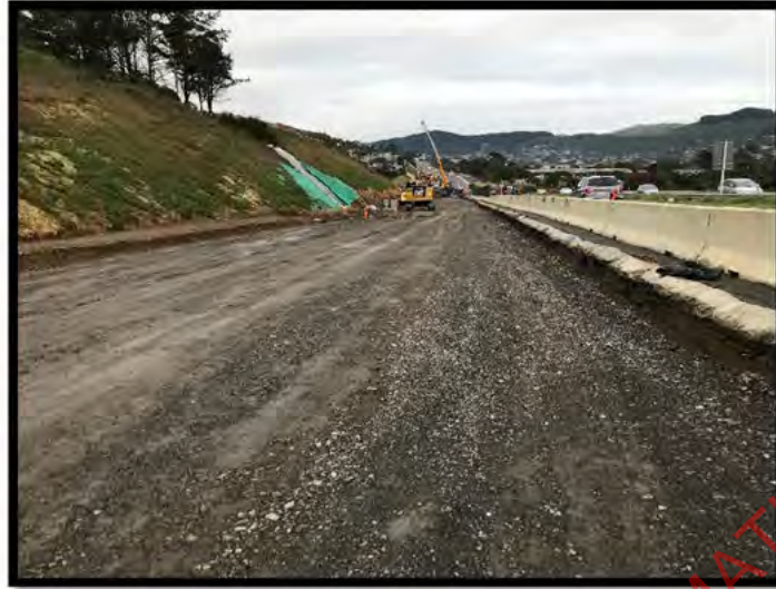
Photo Above: Cut 45 - Construction Platform
