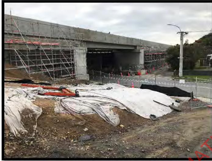
Photo Above: Bridge 26 - Completed bridge structure and Barrier Installation complete
