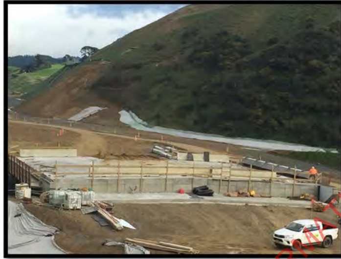
Photo Above: BR6 - Bridge deck
