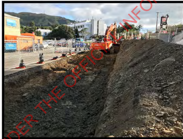
Photo Above: RW7 Undercut commenced
