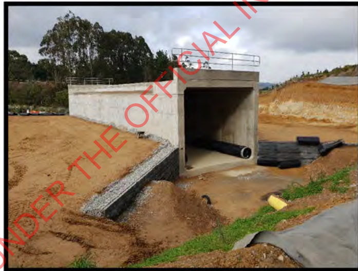
Photo Above: Bridge 12
