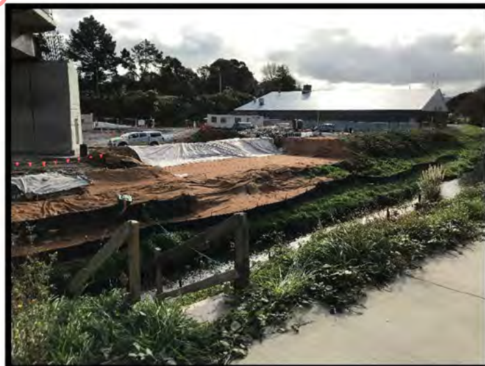
Photo Above: RW9 Undercut commenced
