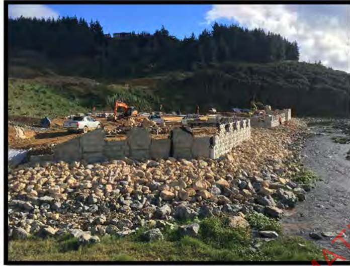
Photo Above: Rip Rap around MSE
