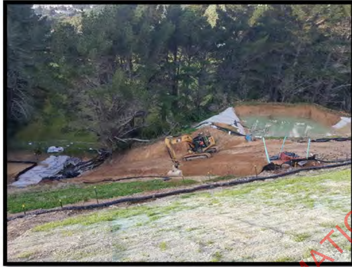
Photo Above: Fill 37C Batter Works
