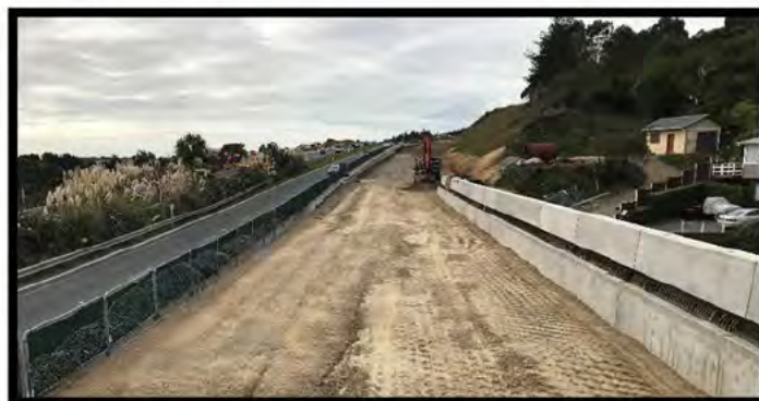
Photo Above: Bridge 26 - Northern Approach Embankment Construction
