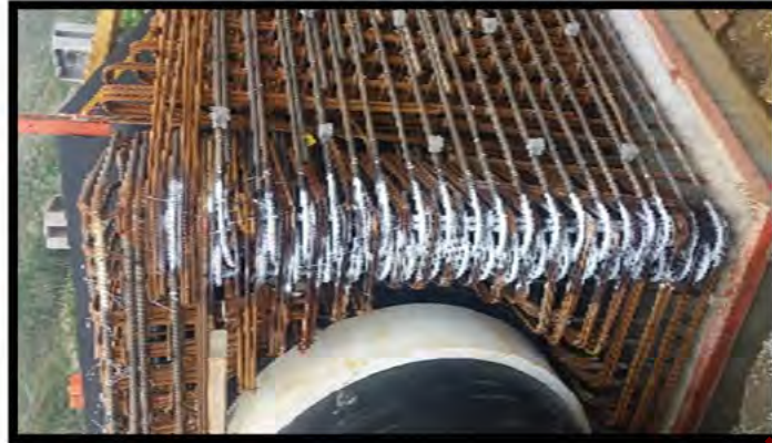
Photo Above: 9040 Culvert
