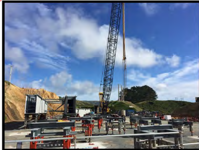
Photo Above: Bridge 20 launch yard
