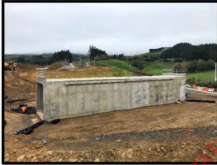
Photo Above: Bridge 12
