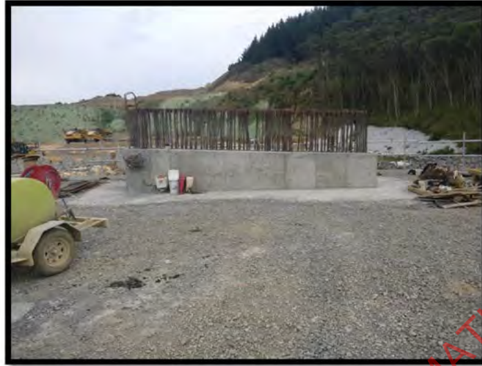
Photo Above: Bridge 14 – Abutment A – Abutment Beam
