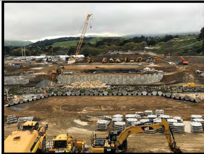
Photo Above: Bridge 15
