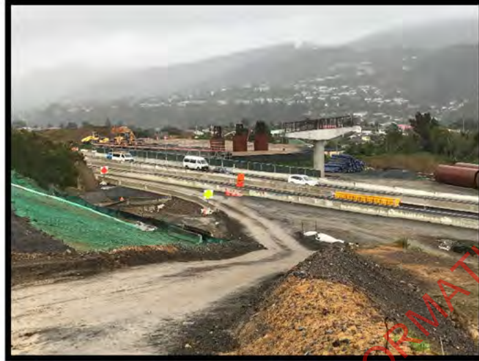
Photo Above: Bridge 25 – Abutment A RSE Construction
