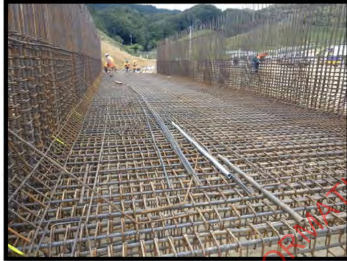
Photo Above: Bridge 11 base slab
