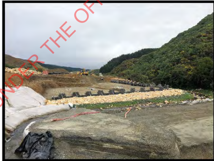
Photo Above: Bridge 4 south
