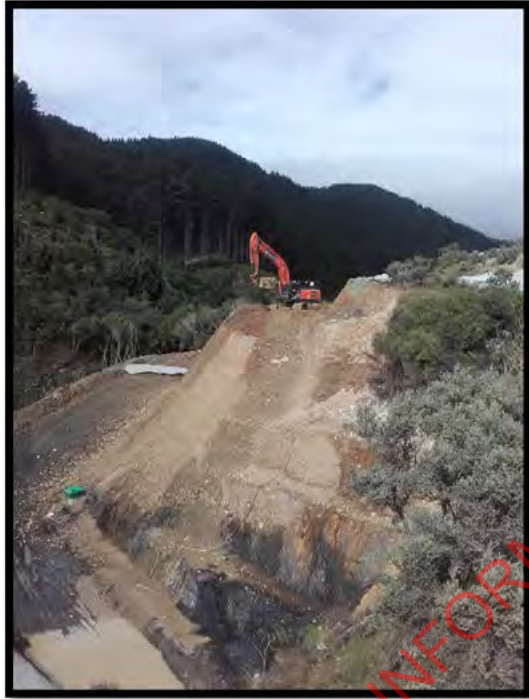
Photo Above: B1 Bridge 3 North Excavation
