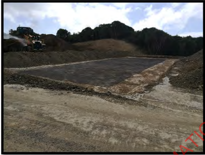
Photo Above: Fill 40 Cut – Fill Transition
