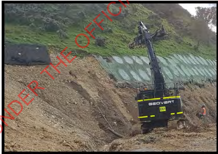
Photo Above: B1 Cut 3.01 Soil Nail Installation.
