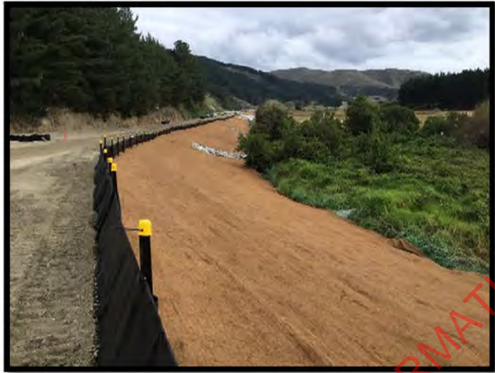
Photo Above: A1 Coast Rd batter stabilisation
