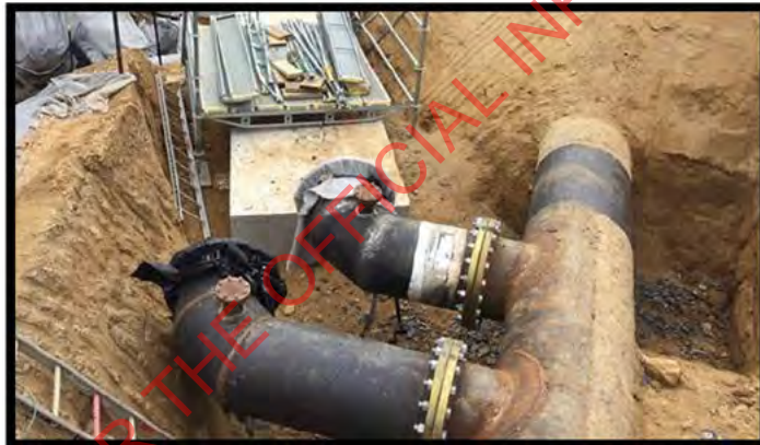
Photos Above: Spools installed for the Br19 temporary water relocation to tie in to 2
