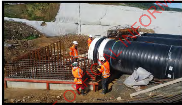
Photo Above: 9040 Culvert
