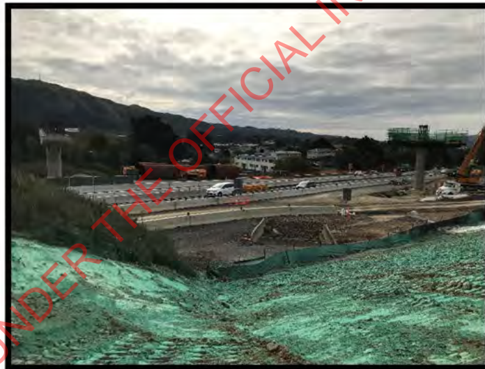
Photo Above: Bridge 25 headstock construction
