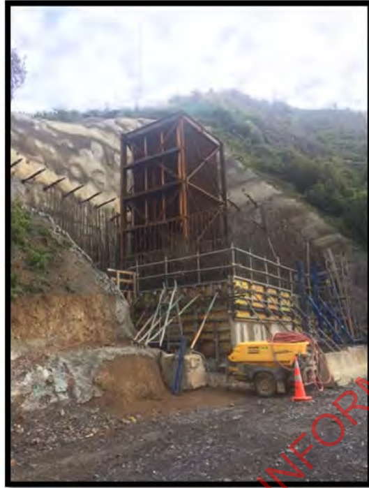
Photo Above: Bridge 20 Pier 2
