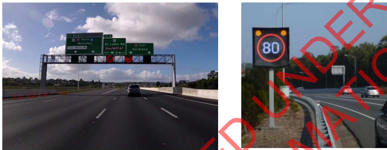
Figure 1: Example of gantry structure and VSLS
