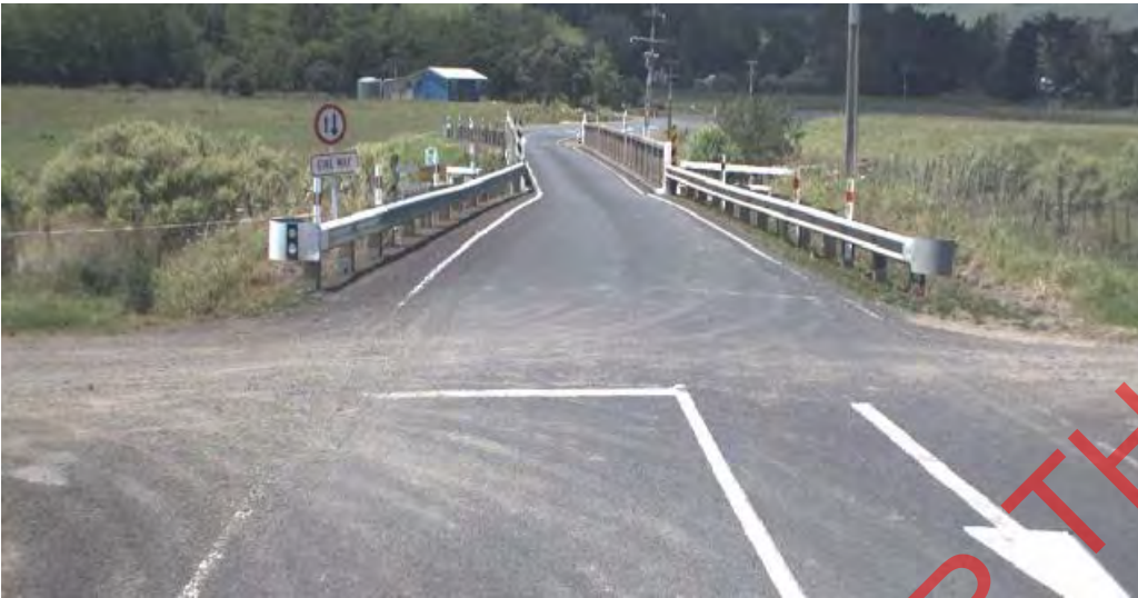
Waimamaku River (Lowes) Bridge
