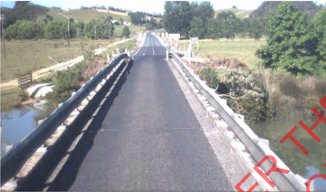
View looking west over Kaeo Bridge
