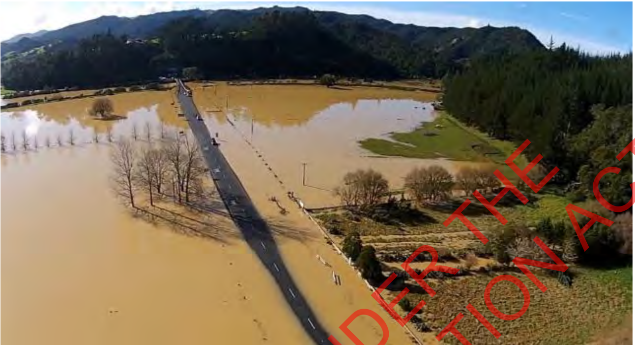
Photograph looking east toward the one lane bridge.
