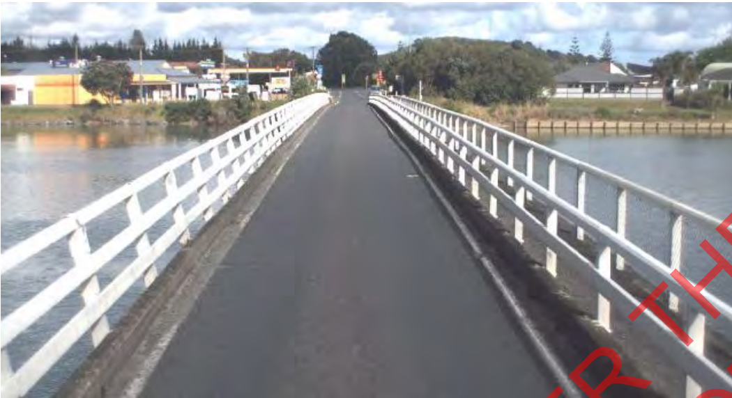
View looking north over Taipa Bridge
