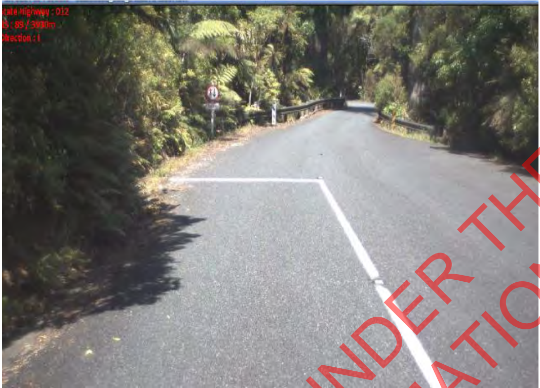
View looking north toward the bridge
