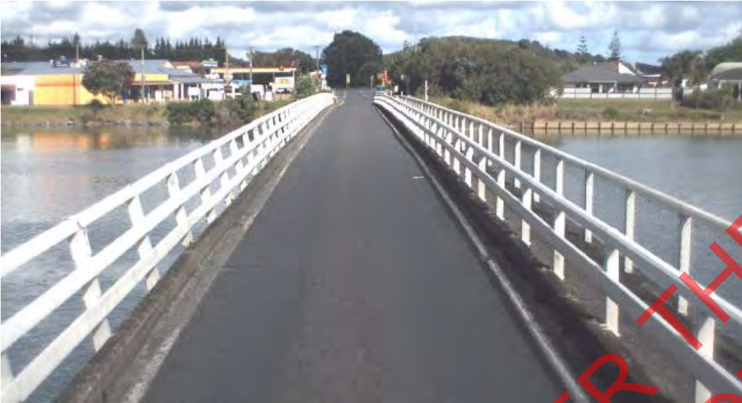
View looking north over Taipa Bridge
