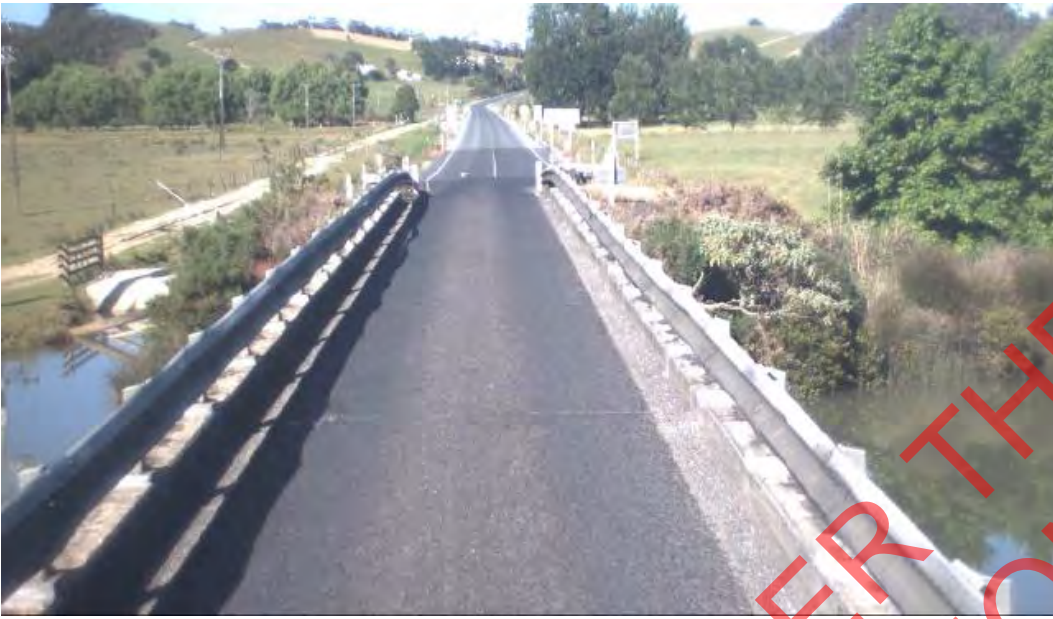
View looking west over Kaeo Bridge
