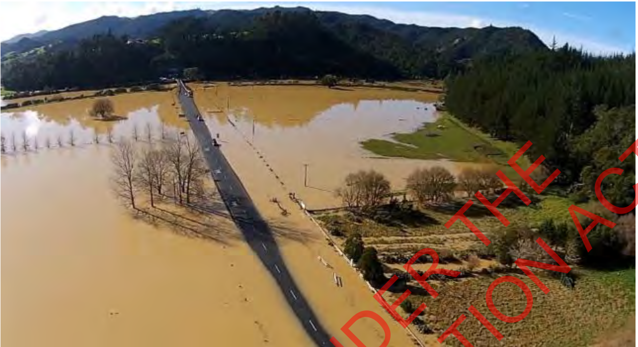
Photograph looking east toward the one lane bridge.
