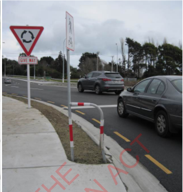
Photo 11 – Damaged holding rail
