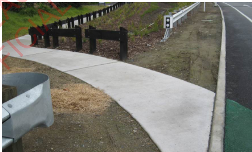
Photo 5 – Low fence/barrier at cycle exit from southbound approach
