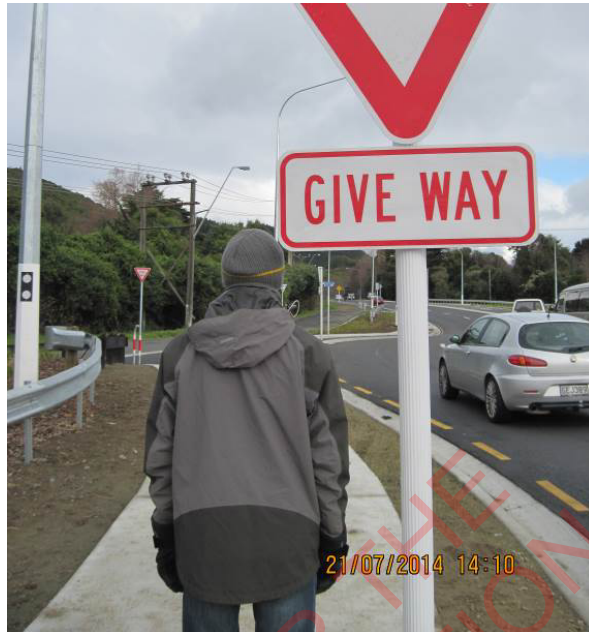
Photo 15 – Low mounting of supplementary sign
