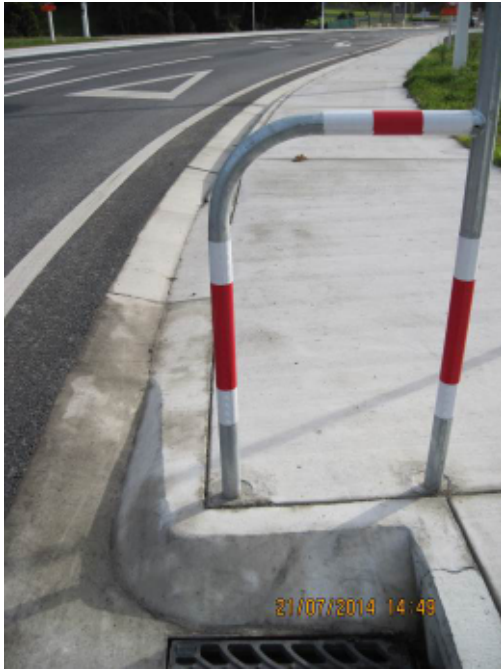
Photo 10 – Holding rail at kerb
