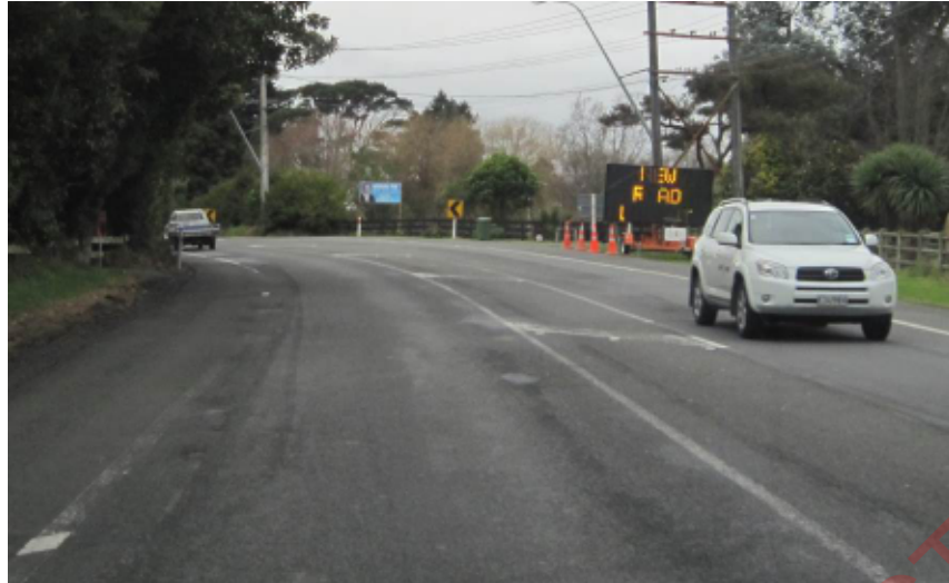
Photo 3 – Curve on northbound approach prior to roundabout
