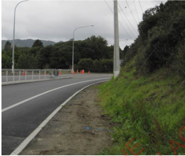
Photo 2 – Concrete power pole on the inside of the southbound approach curve
