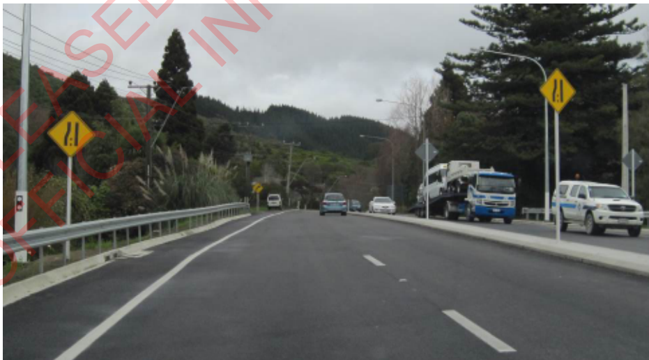
Photo 14 – Right hand side PW-43.3 mounted higher than left hand side
