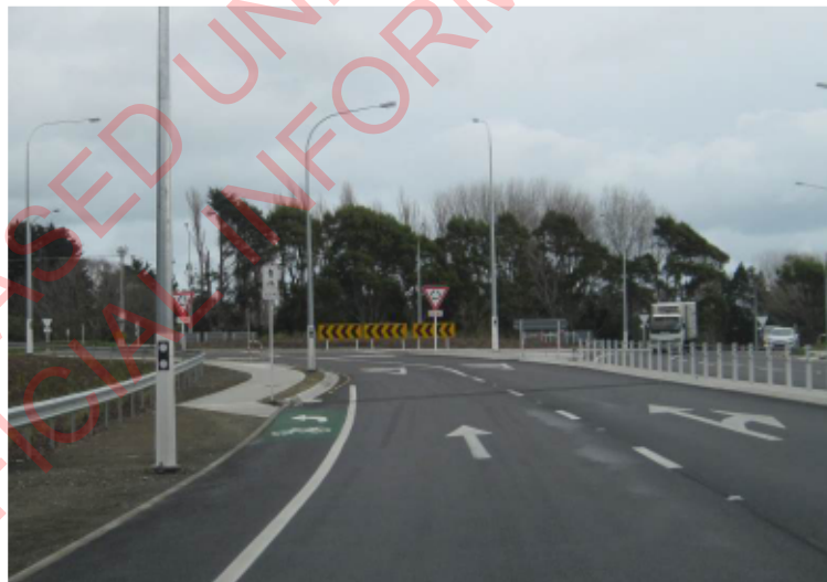
Photo 7 – Second southbound cycle exit
