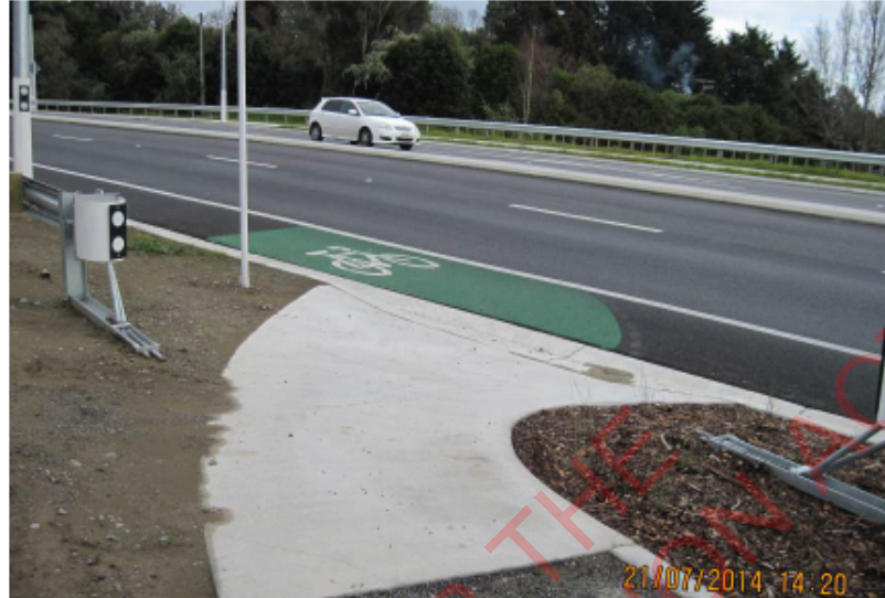
Photo 12 – Cycle exit southbound onto SH1
