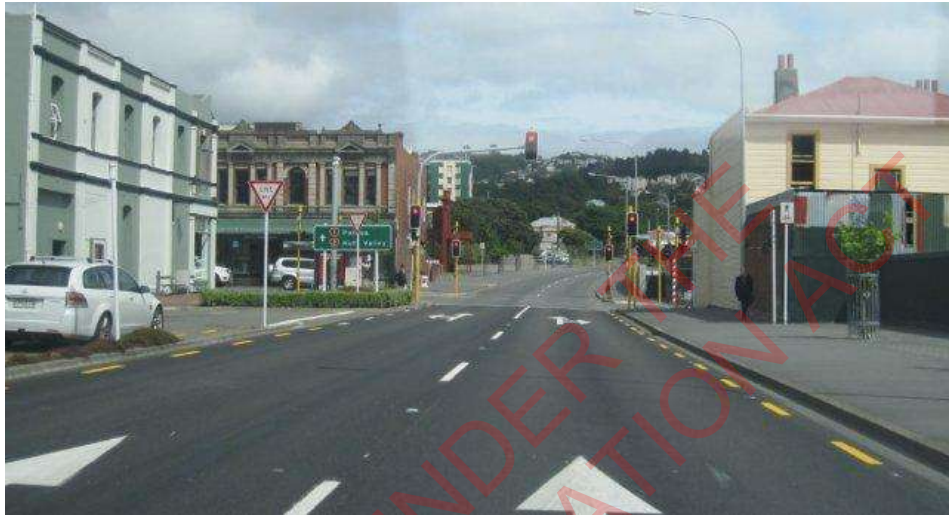
Photo 1 – Karo Drive approaching Cuba Street
